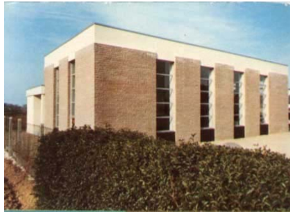
Fig 3. West Exchange, Jersey
